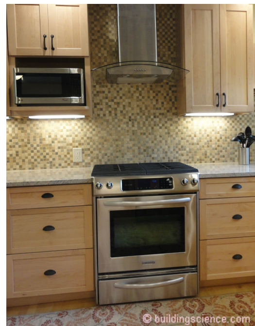
Photograph 4: Kitchen Range Hoods - Exhaust systems such as kitchen range hoods can lead to significant negative pressures.
